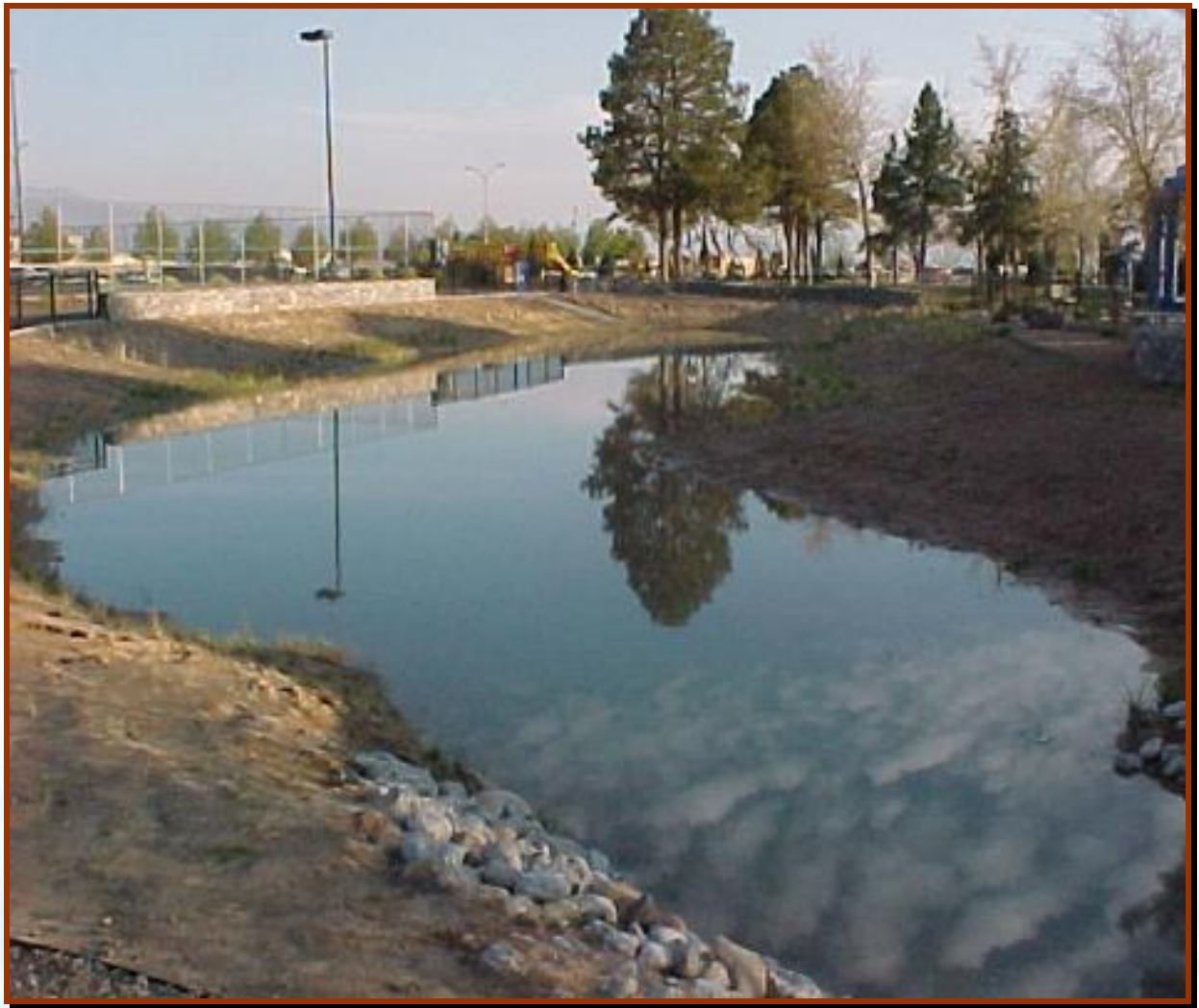
Roskos Field Pond at Haynes Park in Rio Rancho was built in cooperation with the City to control storm water run-off. Gambusia fish have been placed in the pond to control mosquitoes
