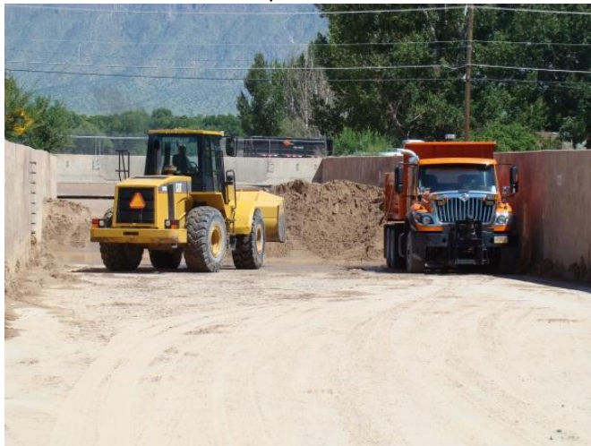
Figure 9: 2010 – Sediment removal upstream of Corrales Road bridge
