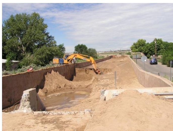
Figure 7: 2006 – Post storm sediment removal at Corrales Road bridge
