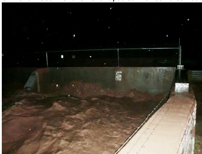
Figure 10: 2013 – Hydraulic Jump into Corrales Road bridge
