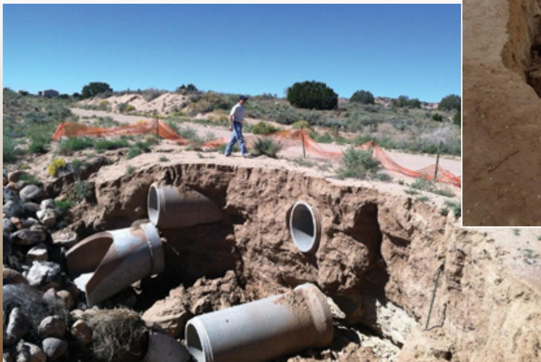
**Arroyo movement can also expose large underground water and sewer pipelines and result in outages of vital services.**
