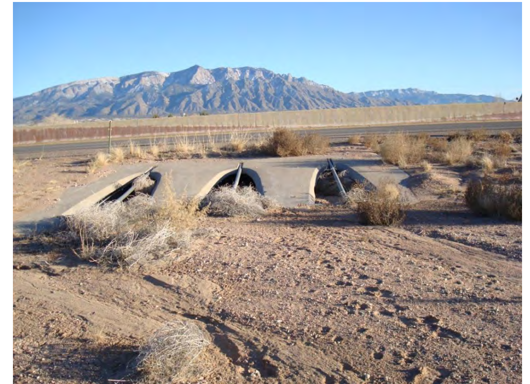
Photo 15: Crossing WC_04X (3 – 60” CMP, capacity ≈ 422 cfs)
