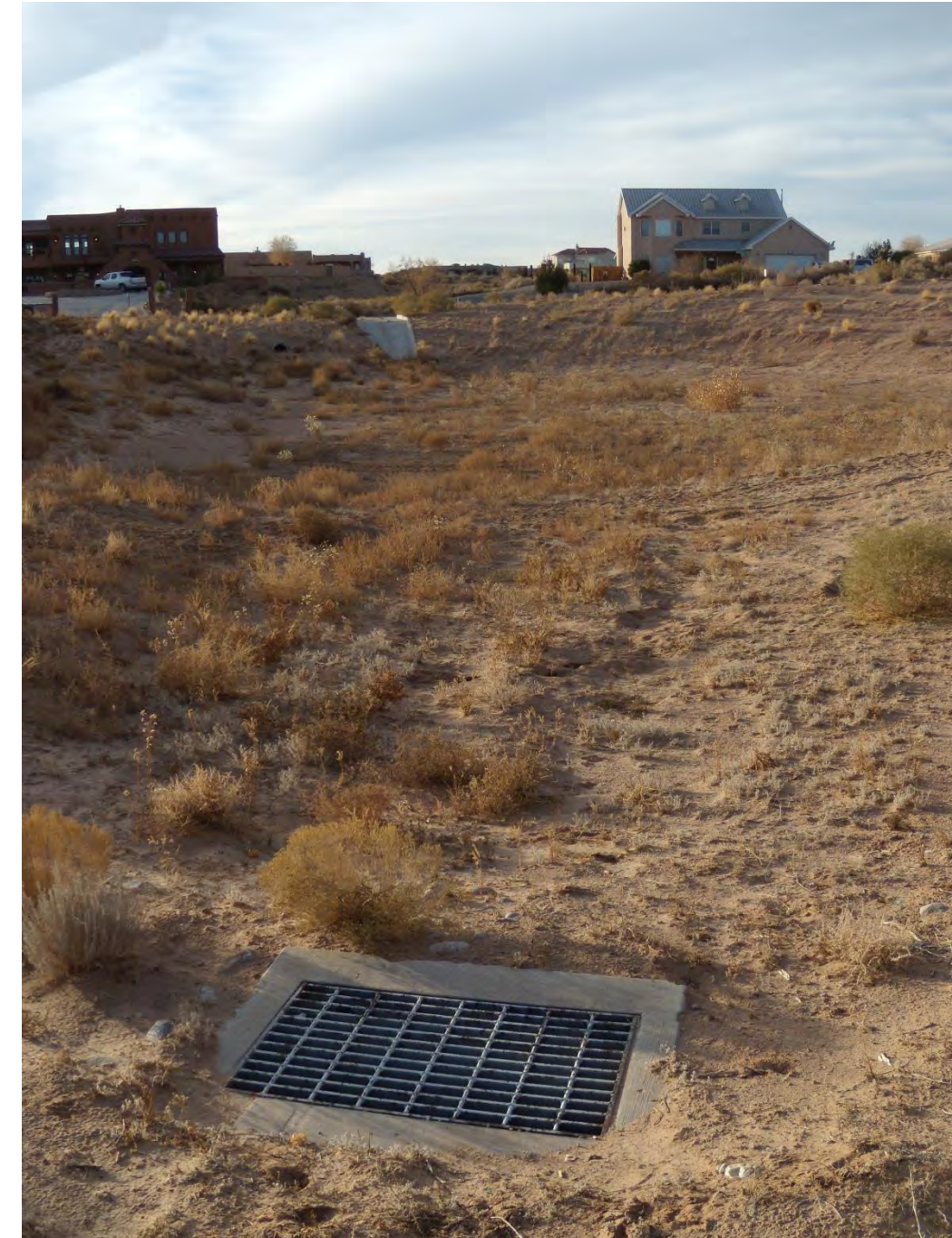
Photo 21: Christopher Pointe Pond (WC_06P), with the outlet structure visible in the foreground.
