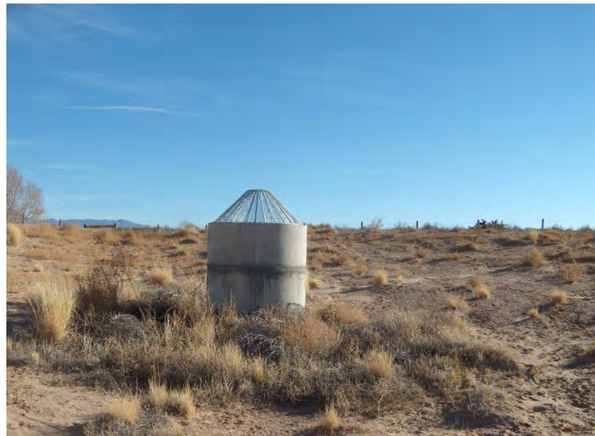
Photo 8: Pond # 2 outlet structure is a concrete riser pipe without ports.
