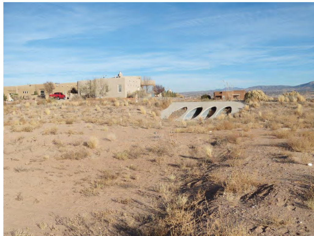
Photo 4: Pond # 10 (WC_03P, capacity \approx 4 AF); culvert crossing serves as outlet structure.
