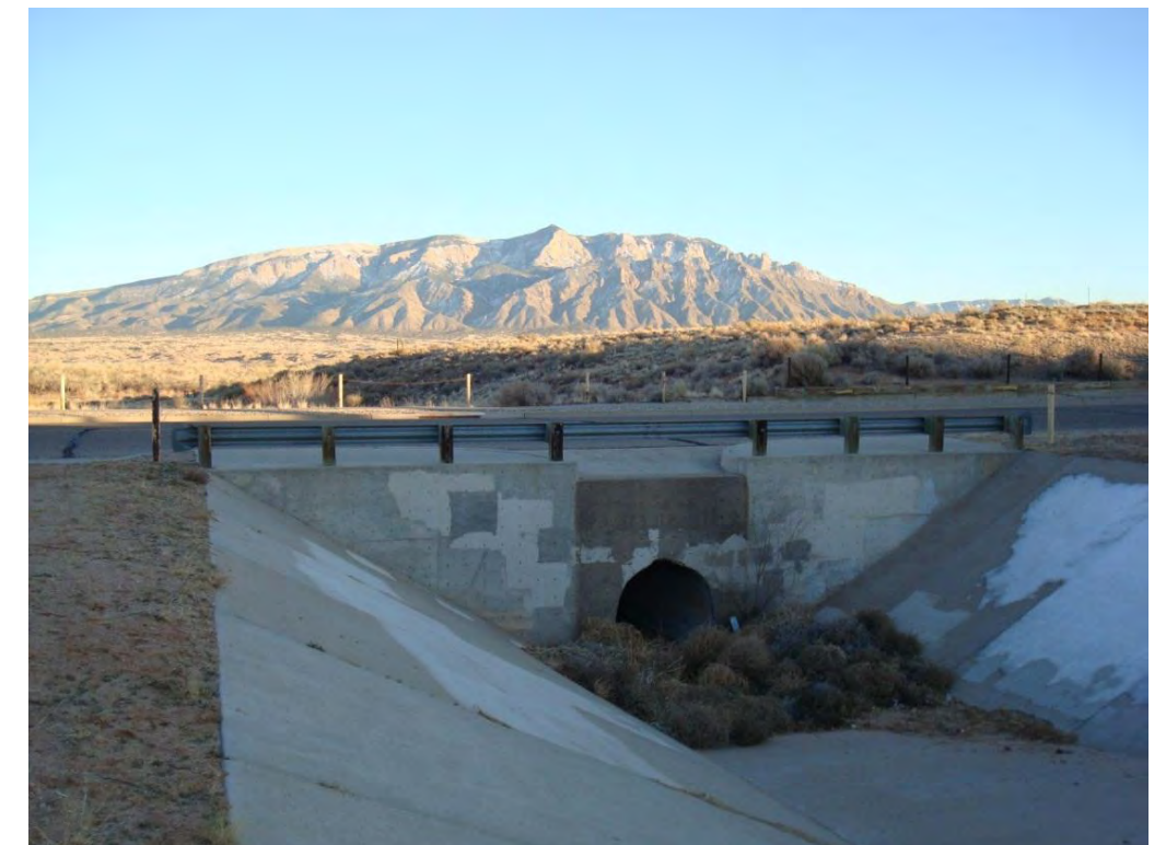
17: Culvert at Willow Creek Road and Basin B (1 – 72” CMP, capacity ≈ 355 cfs)
