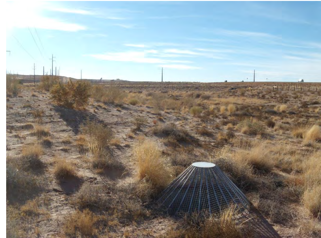
Photo 1: Pond # 13 (WC_01P, capacity ≈ 3 AF), looking west from the outlet.
