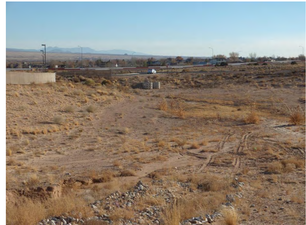
Photo 5: Sandoval County Pond (WC_04P, capacity \approx 9 AF), with ported riser outlet structure in the background.
