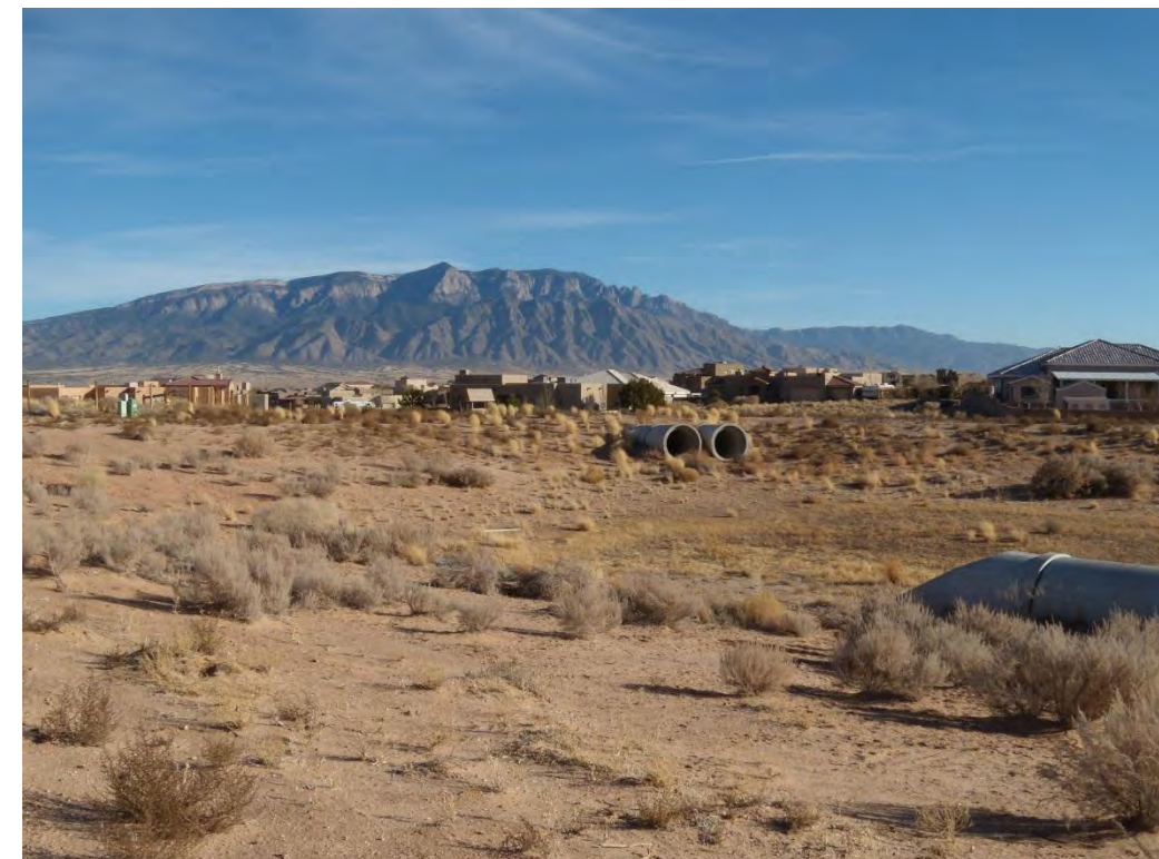
Photo 2: Pond # 6 (WC_05P, capacity ≈ 3 AF), with the outlet visible in the background.
