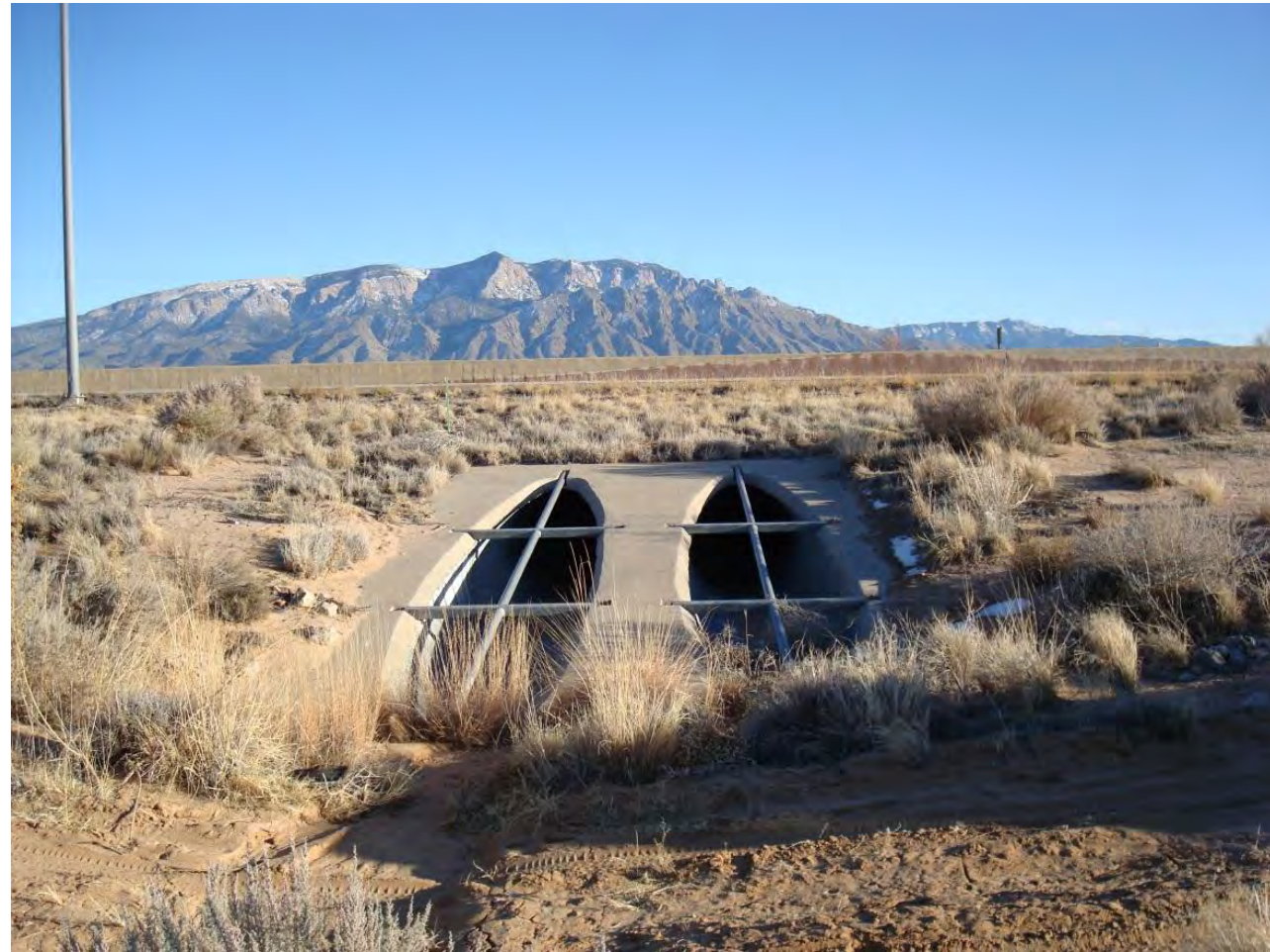
Photo 13: Culverts at NM 528 and Basin A (2 –60” CMP, capacity ≈ 335 cfs)
