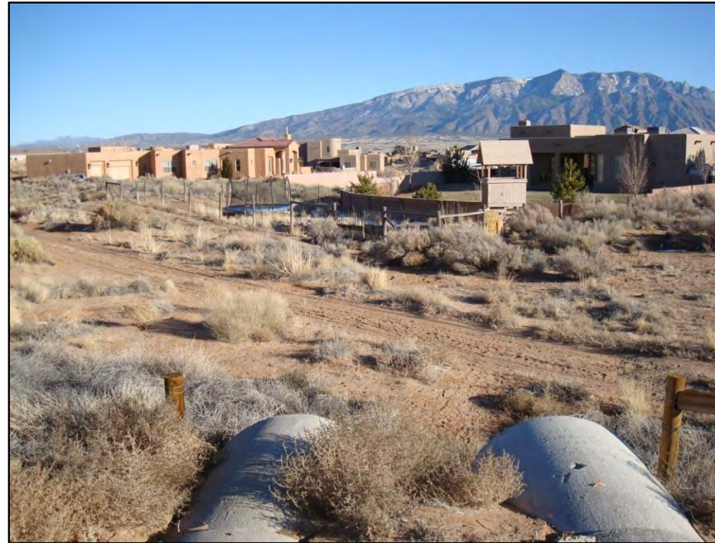
Photo 9: Home located in former flow path of Arroyo, looking east from SAD 6 Pond # 6; the outlet structure of the pond (two reinforced concrete pipes) can be seen at the bottom of the photo.
