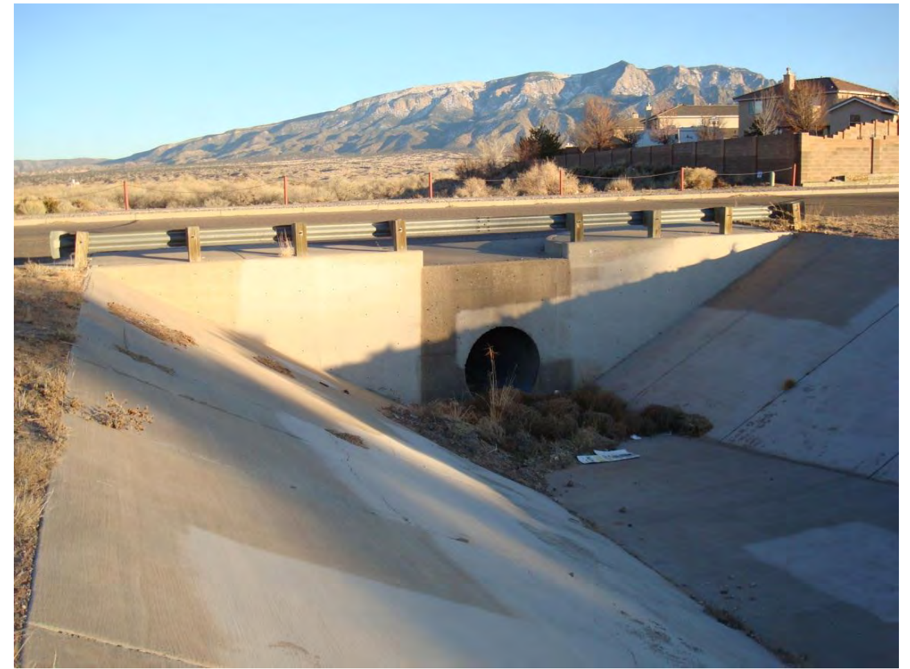
Photo 14: Culvert at Willow Creek Road and Basin A (1 –66” CMP, capacity ≈ 290 cfs)
