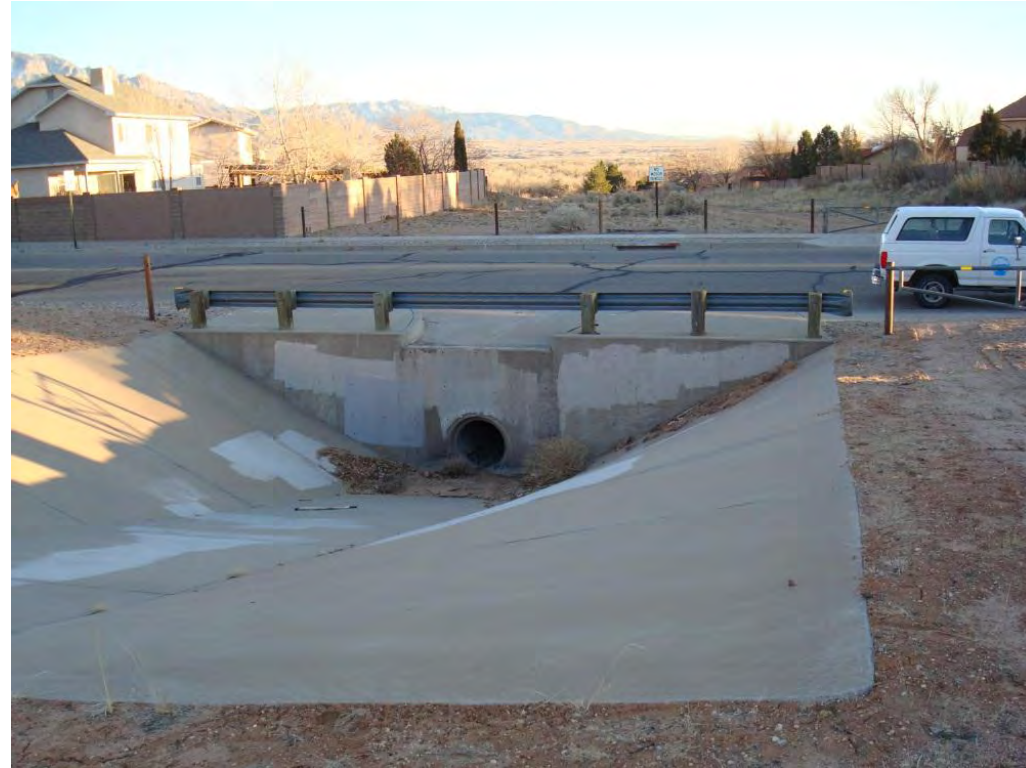
Photo 19: Storm drain inlet at Willow Creek Road in Basin C (36" RCP, capacity \approx 90 cfs).
