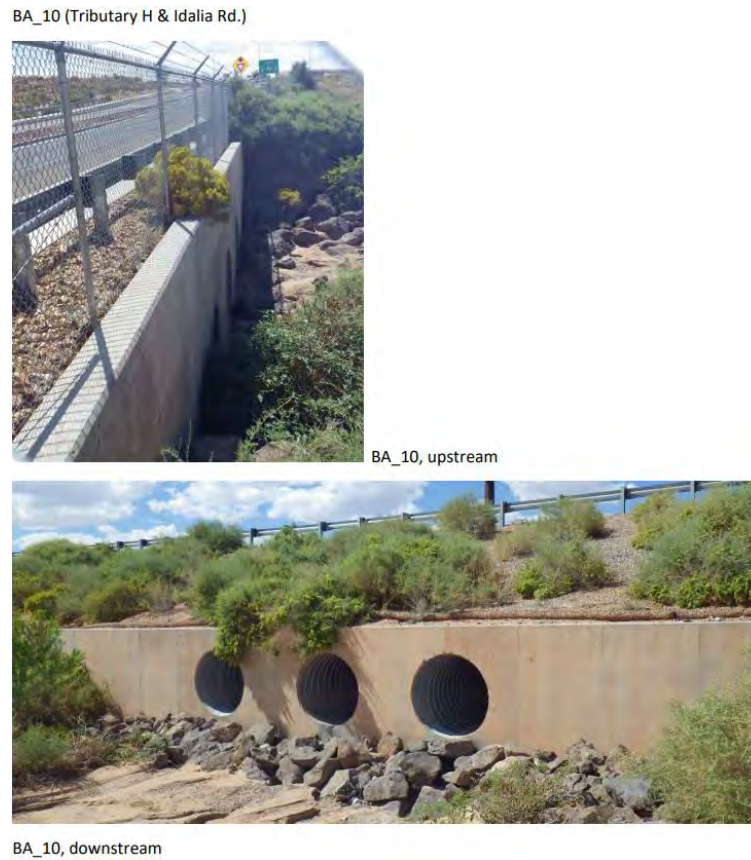
Figure 1: Structure BA_10, photos provided by SSCAFCA
