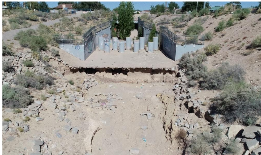
Figure 6: Loss of Sediment in a Degraded Channel
