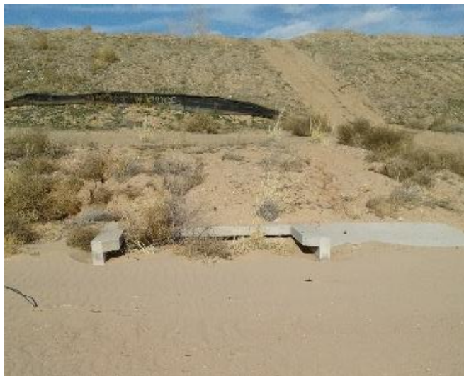
Figure 5: Buried Energy Dissipator in an Aggraded Channel
