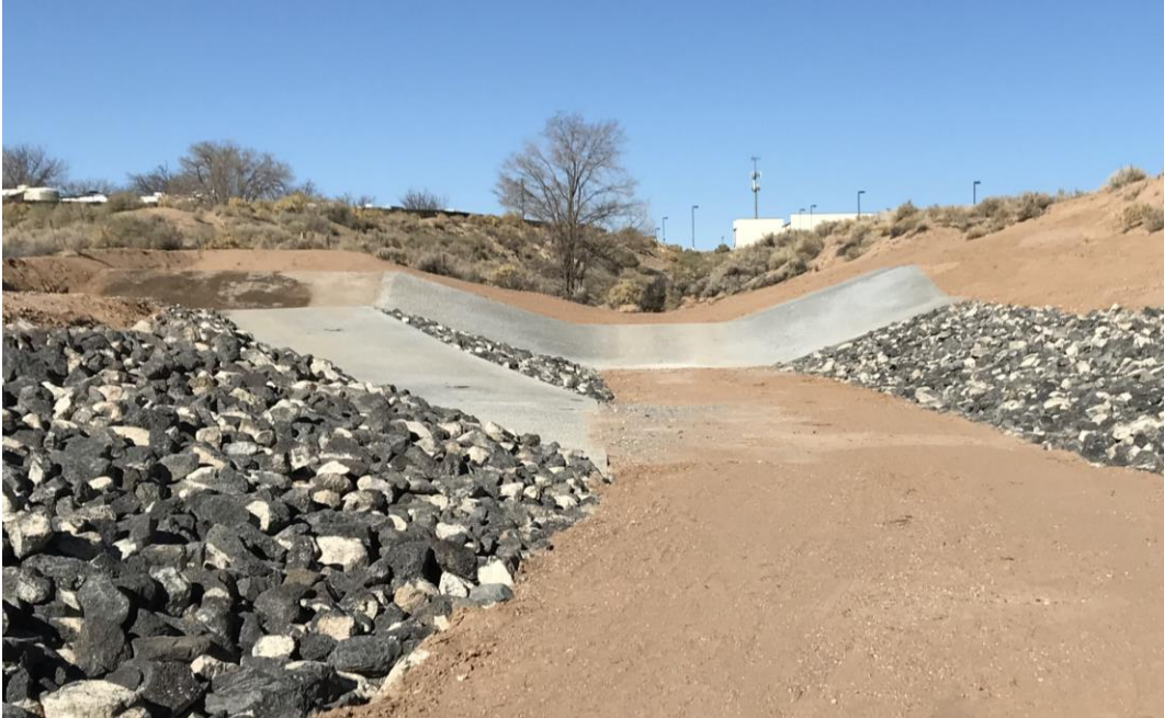
Figure 3: Maintenance Access Road & Ramp Configuration.
